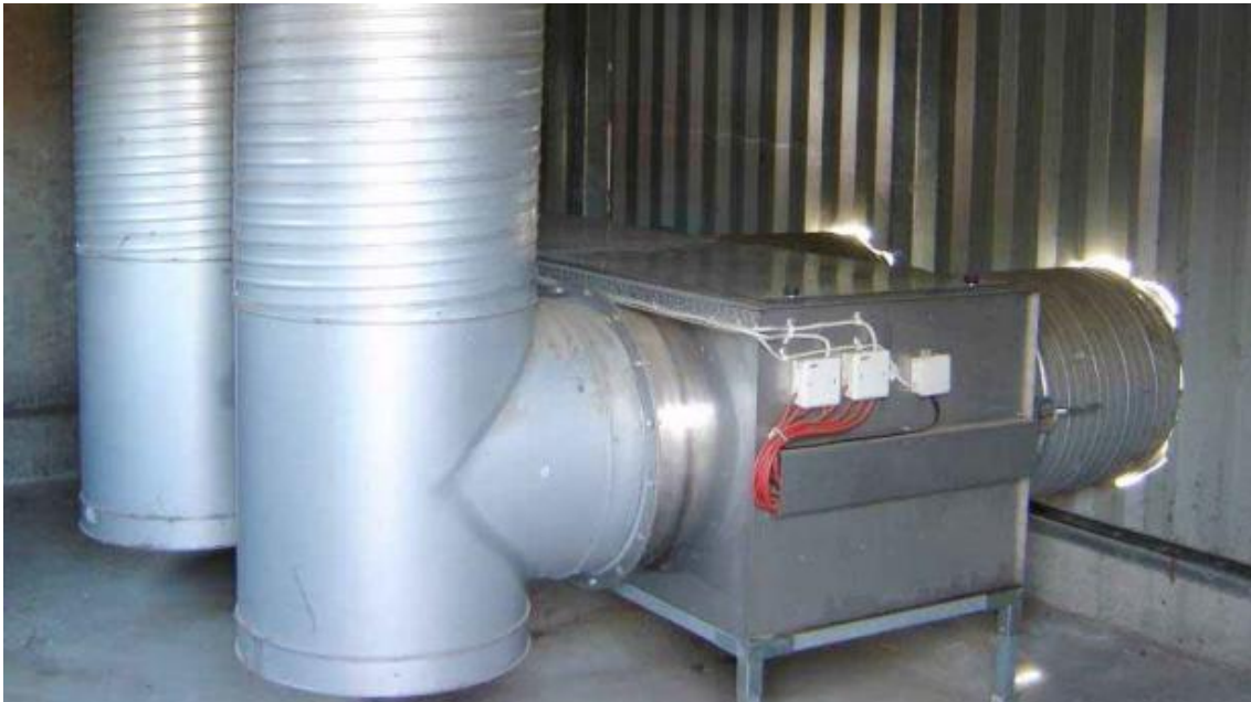
Figure 5. Ozone treatment for ventilation air (Photo: Swedish Waste Mgmt Assoc)
