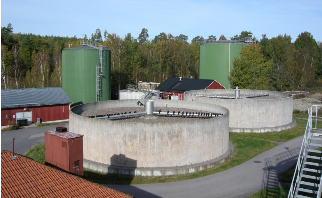
Figure 1. Anaerobic digestion plant where different organic waste fractions are processed (Vimmerby Energy Company).
