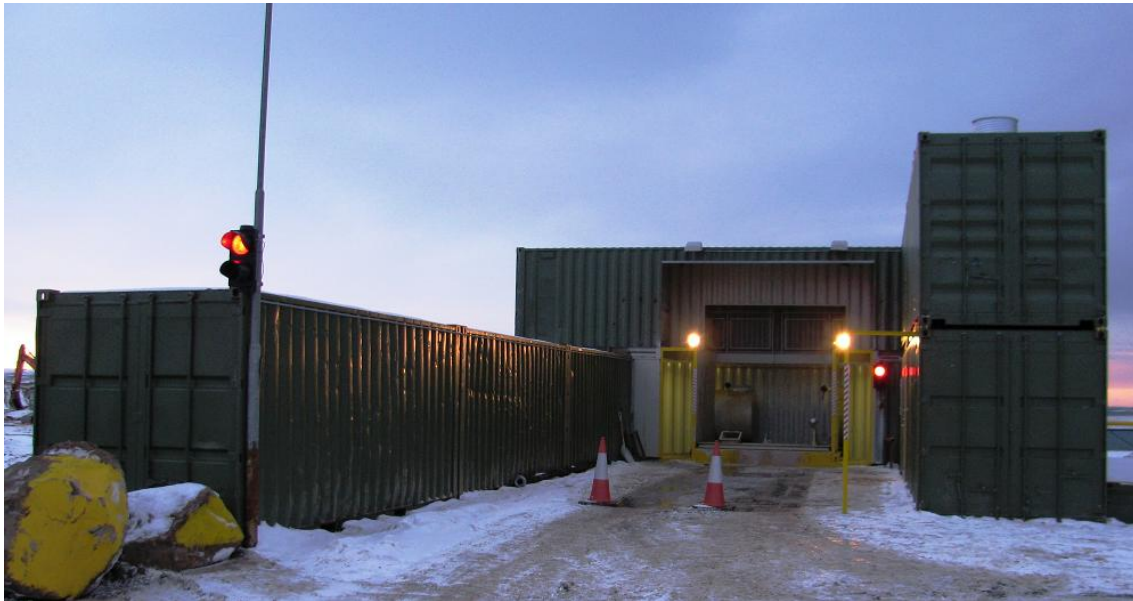
Figure 14 Receiving station for liquid and odorous material – hook up for pumpable waste and a hatch for receiving solid material
