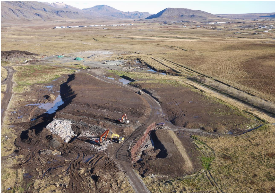
Figure 11 Overview of the current landfill site for baled household waste.
