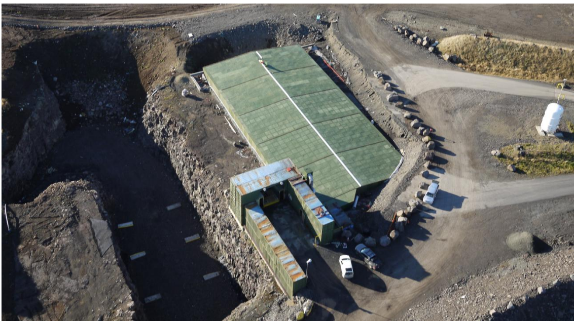
Figure 13 Receiving station for liquid fractions and odorous solid material, covered by a roof of steel and timber.
