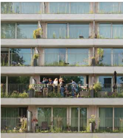
Horizontality of the facade with a strong indoor-outdoor connection.
