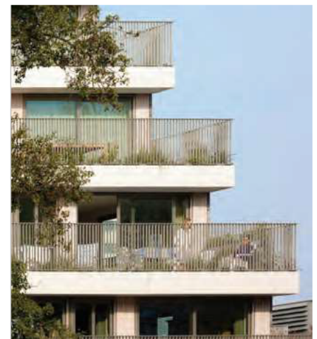
Horizontality of the facade with a strong indoor-outdoor connection.
