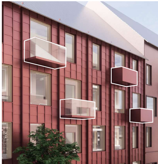
Closed solid railing or glass railing with no articulation. Flat appearance
