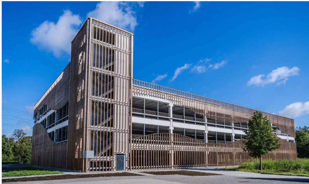
Image 5.3: Multistorey car park in Limburg, Netherlands Prefabricated timber units, generous ceiling height and a movable central ramp make it easy to later convert the building into, for example, classrooms, workshops or an event space.
