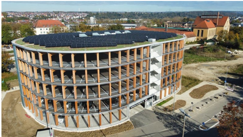
Image 5.2: The Holzparkhaus Wendlingen car park is built from prefabricated timber units, which make it possible to convert the building or disassemble it.
